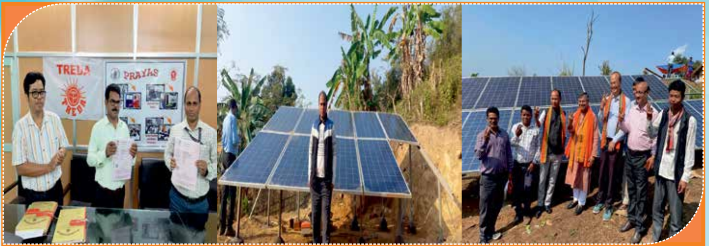
Supply & Installation of 1 No. Solar Powered Community Water Purification (RO) Plant at Datta Molsom Para ADC village in Teliamura under Khowai District Tripura.
