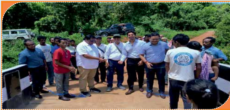
Construction of Culvert over Umsohpeing River (Umsning C & RD Block) Ri-Bhoi, Meghalaya.
