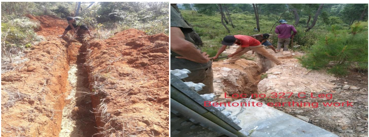
Fig 2C- Bentonite Earthing
